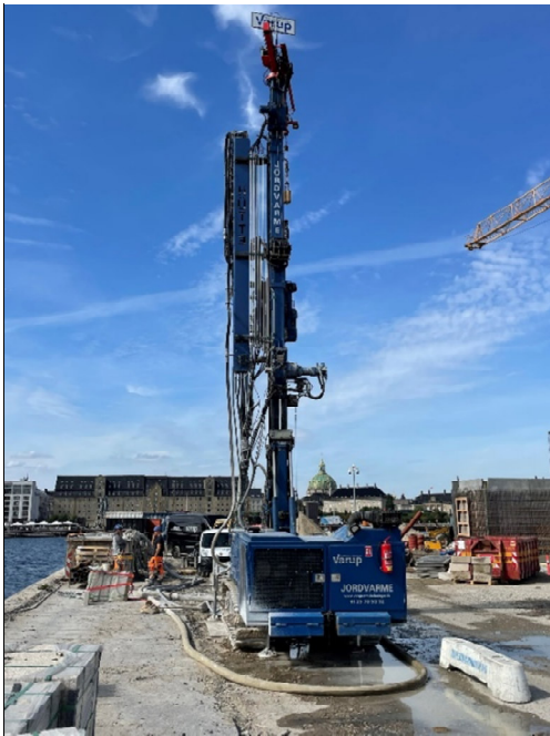
Image 3: Drilling rig Photo: Varup
